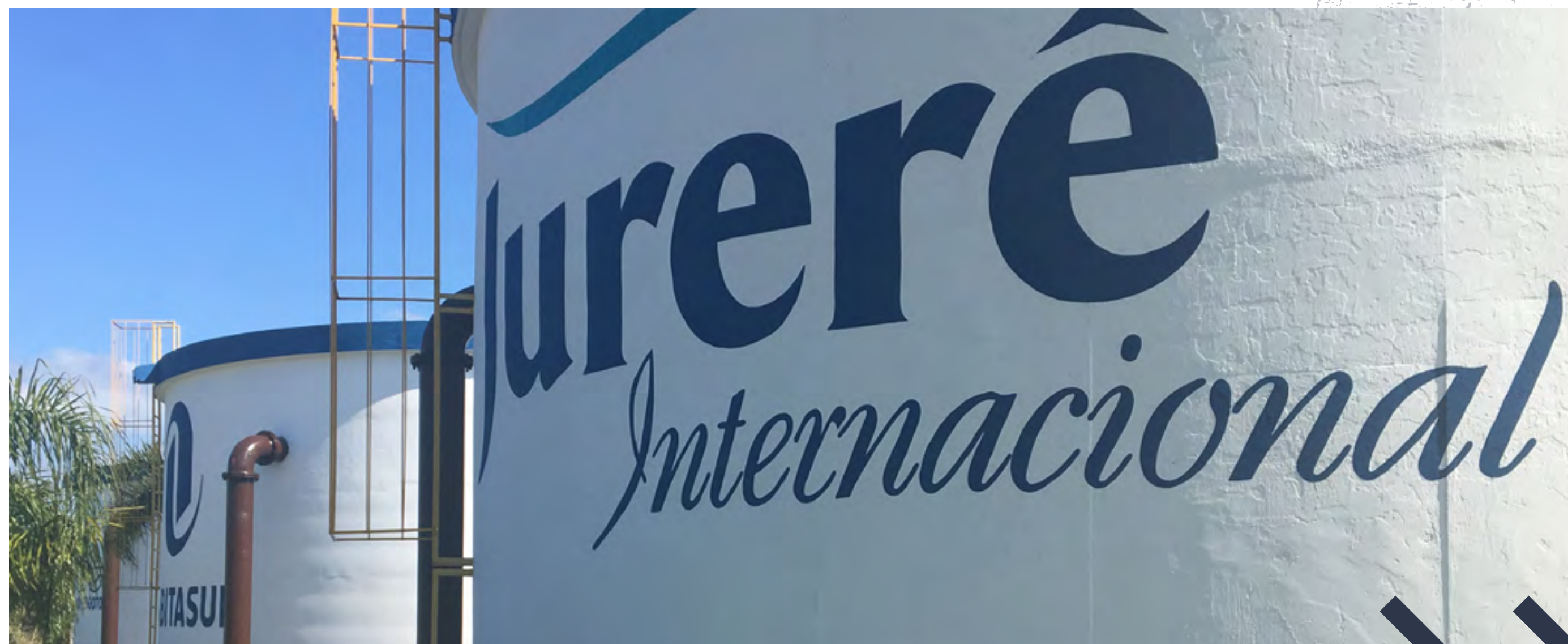
Reservatório SAE (Reservoir of the Water and Sewage System) – Jurerê Internacional/SC
