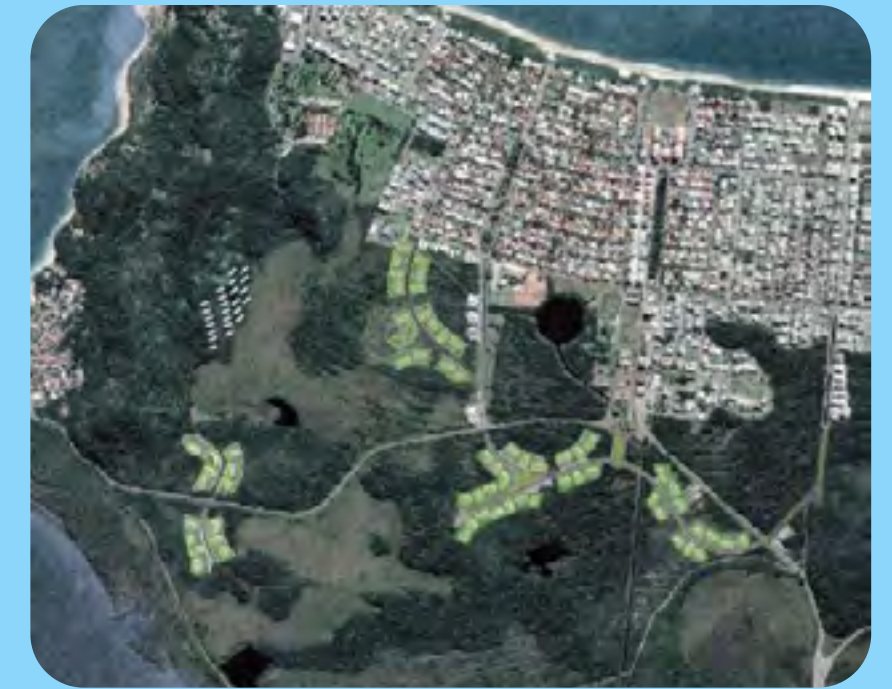
Review of environmental studies and urban studies for the area of special urbanization
